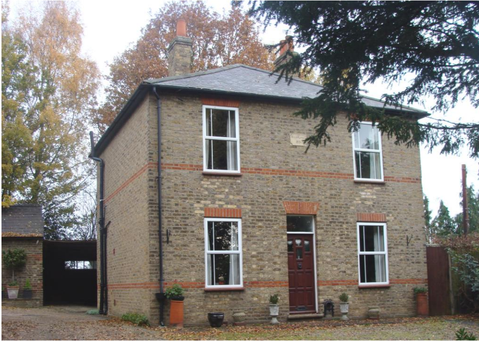
Picture 12. Wesley Cottage, a simple late 19 th century building of charm that despite modern windows (whose impact is reduced virtue of all being of same design) adds to the character of this part of the Conservation Area.
