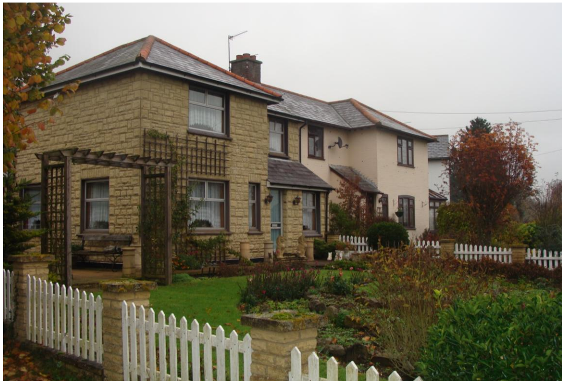
Pictures 26. The front elevations of selected properties at Hillside Cottages have been much changed and altered and are not considered to be of sufficient architectural or historic interest to remain within the Conservation Area.
