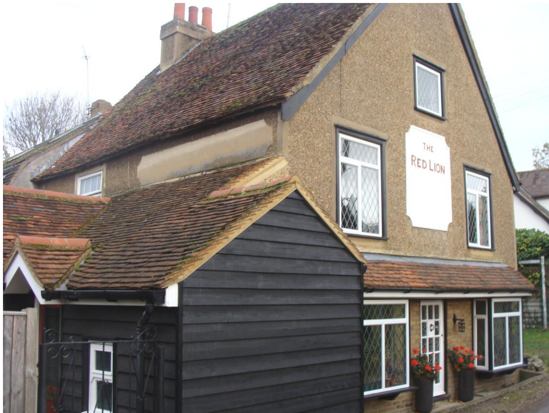
Picture 16. The former Red Lion PH. Its general mass and particularly its steeply sloping roof contribute to the street scene despite subservient extensions to side and other detailing.
