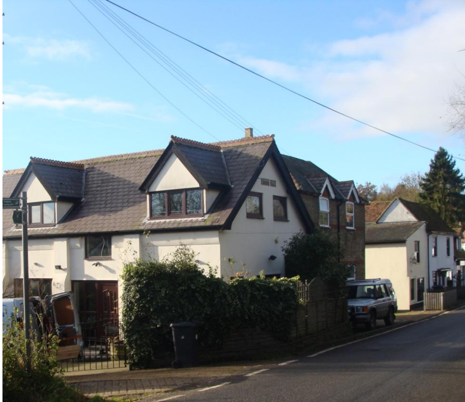
Picture 2. The former Ebenezer Temperance Hall, now altered to a degree that its original architectural and consequently historical importance is much reduced. Now rendered, entrance detail and railings removed, new dormers, new windows.
